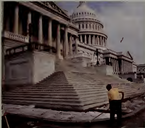
Repairs to sidewalk on the East Front of Capitol.
